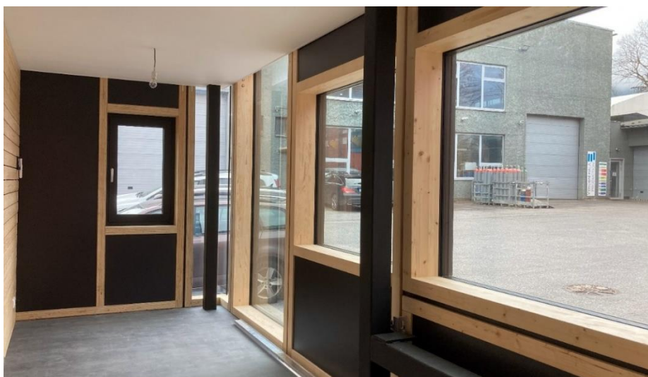
Fig. 22. Interior view of the wooden lab with different timber curtain wall units.
