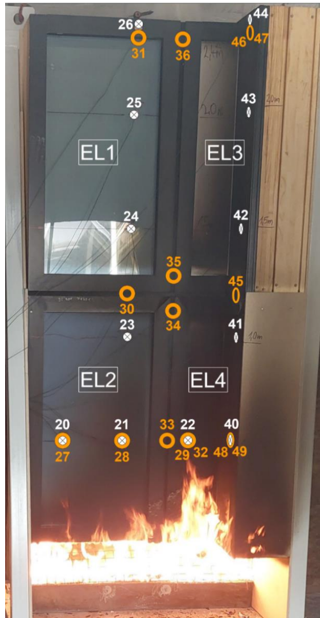
Fig. 10. The specimen of the timber curtain wall during the 46 th minute of the fire test. The marking of thermocouples and the curtain wall units were added to the photo.
