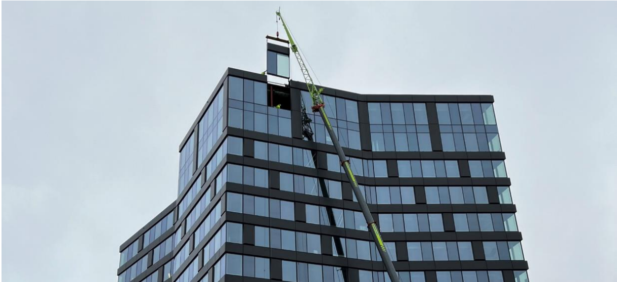
Fig. 1. Photo of a final unitized curtain wall unit being hung.
